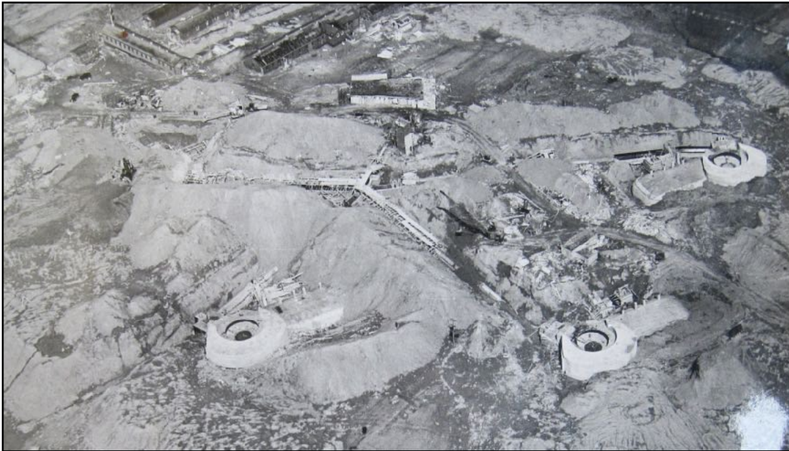
Devils Battery under construction on 8 April 1941. The three concrete emplacements can be seen, as well as the lines of the concrete underground tunnels that linked the emplacements to the main tunnel junction in the centre. The small building just above the junction is the cover for the command post, and is connected to the junction by a short tunnel. The large rectangular concrete structure beside each emplacement is the magazine, with the ground level entrance being the small square concrete structure that can just be seen behind each magazine. The tunnel connecting to the pump chamber for each emplacement is clearly visible. The construction in the extreme upper left corner to the left of the surface barracks accommodation building is the battery plotting room. Devils Battery Fort Record Book.
