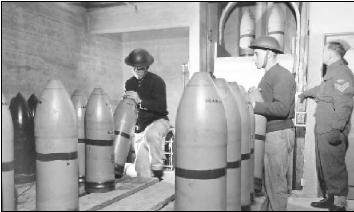
An indication of scale - the projectile room in the magazine, probably at Sandwich Battery early in the Second World War. The hoist to take the shells up to the emplacement floor is in the background. Each shell weighs 380 pounds (178.4 kg). Moving them was not a trivial task. The shells are not fuzed. LAC 399183.
