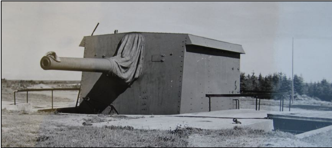
A 9.2-inch Mk 15 gun on Mk 9 mounting at Oxford Battery. Note the extreme simplification of the concrete in the emplacement with no parapet and the lack of an open pit behind the gun. The gun house is completely enclosed. Oxford Battery Fort Record Book.
