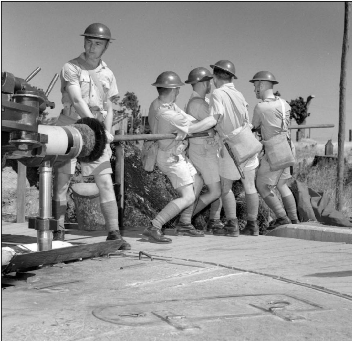
Preparing to ram on a Mk 5 barbette mounting at Albert Head. No. 4 is supporting the head of the rammer-brush-and-sponge against the base of the projectile as others prepare to ram the projectile home. The fuzzy part in front of the brush is the sponge, which was kept wet to ensure that no propellant remnants were smouldering. The projectile is on the rear hoist, seen coming up through the flap doors in the shell pit shield. In this case, four gunners are on the rammer, but three would be more normal. City of Vancouver Archives.
