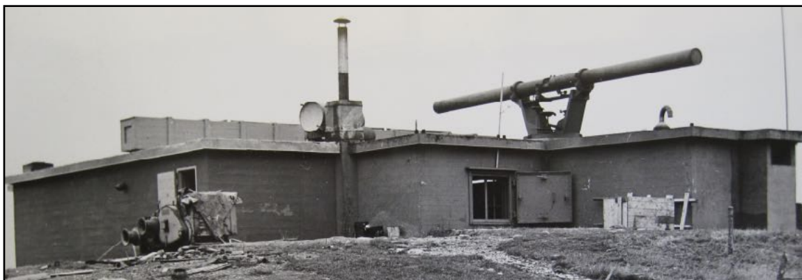
An optical rangefinder (the long rod on the roof) being installed for the 6-inch guns at Lingan Battery at Sydney, NS. The crate is still on the roof of the observation post. The 9.2-inch guns used a similar rangefinder in their battery observation posts. Lingan Fort Record Book.
